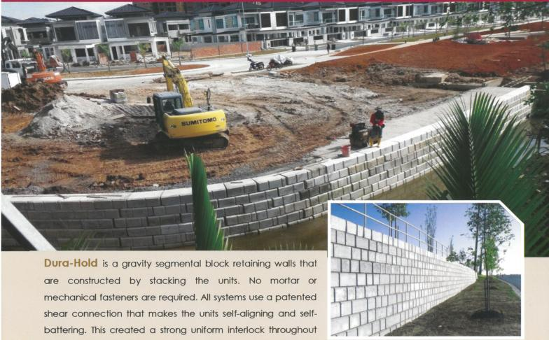
The height of walls built with **Dura-Hold** can be increased substantially when used with Geogrid Soil Reinforcement - please contact our technical support team for more details.
